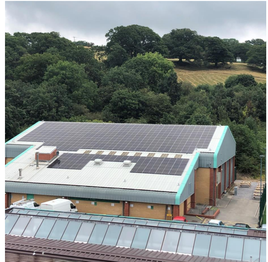
Figure 1.1.1: Solar panels at Ysgol Dinas Bran, Llangollen
